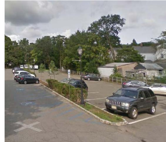
Parking spaces throughout the lot can be converted to porous pavement to capture and infiltrate stormwater runoff from the rest of the parking lot. A preliminary soil assessment suggests that more soil testing would be required before determining the soil's suitability for green infrastructure.
